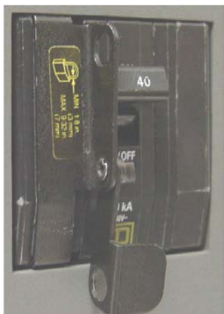
Main Power Disconnect Switch
